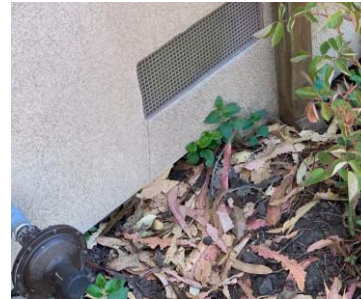
Remove debris next to house
